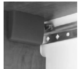
Cover installed over bracket
